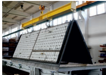
2 Lifting the butterfly formwork Lyft fjärilsformen
