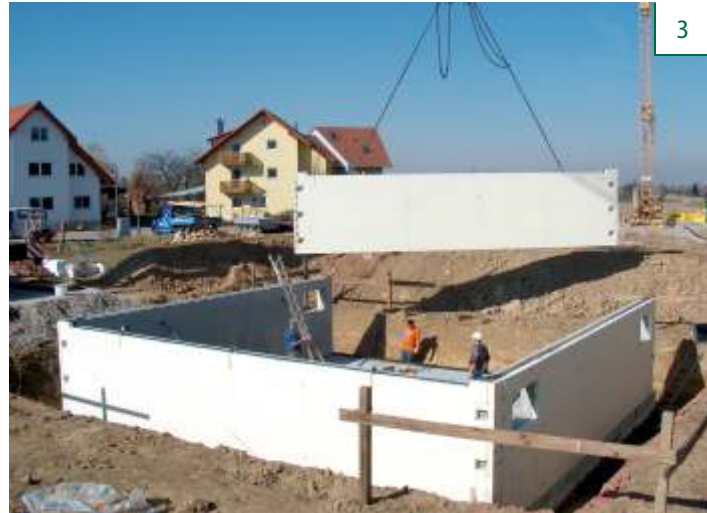
Watertight basement made of massive pre-cast components
