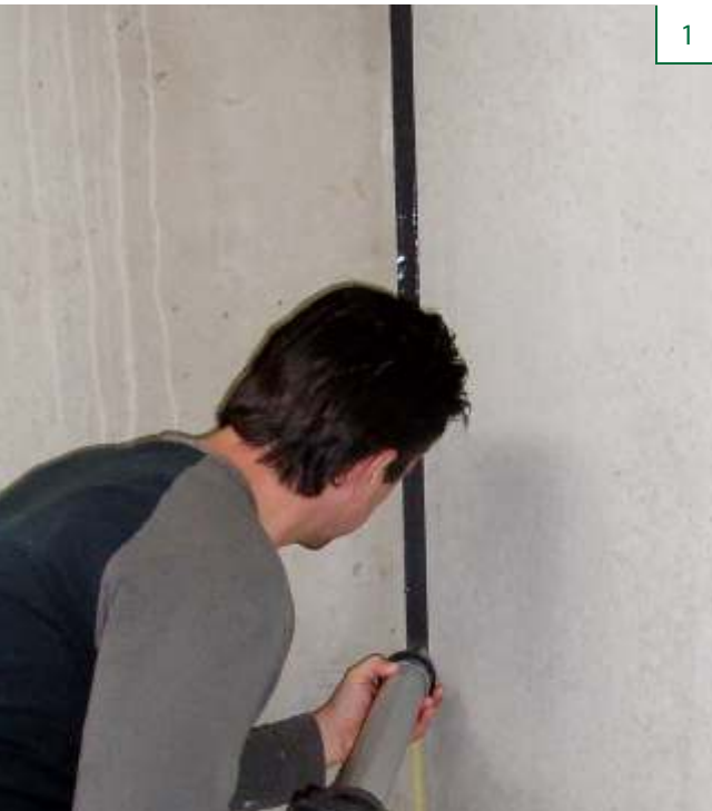
InnoElast® as joint finishing
