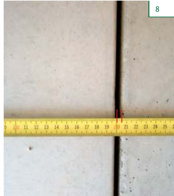
Final joint thickness about 5mm
