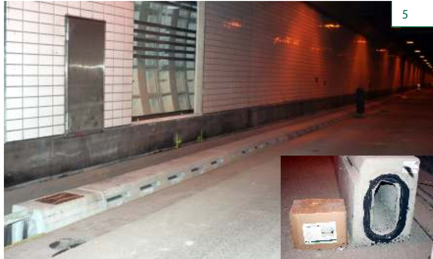
Firm gluing of pre-cast components
