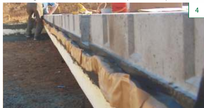
Sealing between bottom slab components
