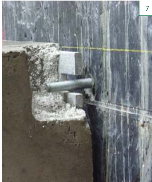
Connection to the existing building
