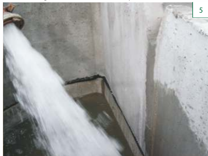
Watertight immediately after application
