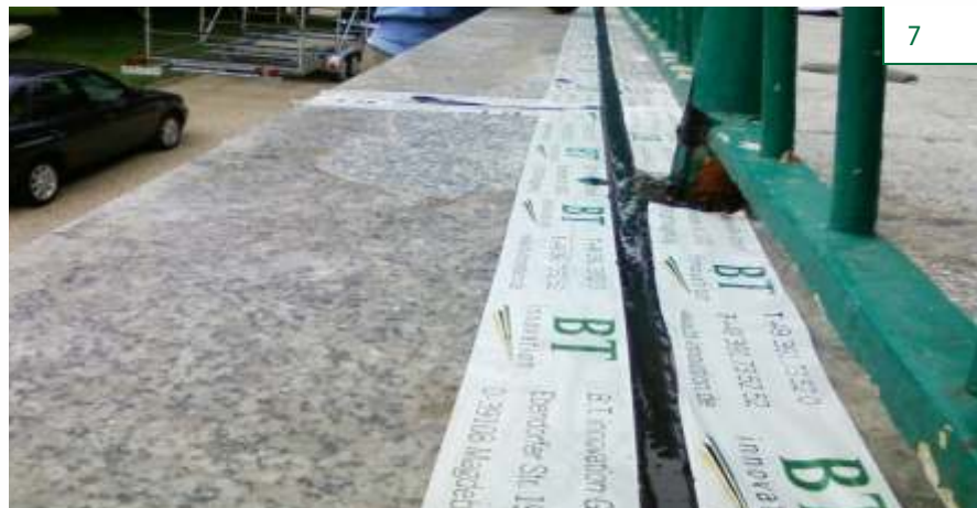
InnoElast® as sealing for floor joints
