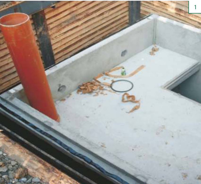
Sealing of shaft joints
