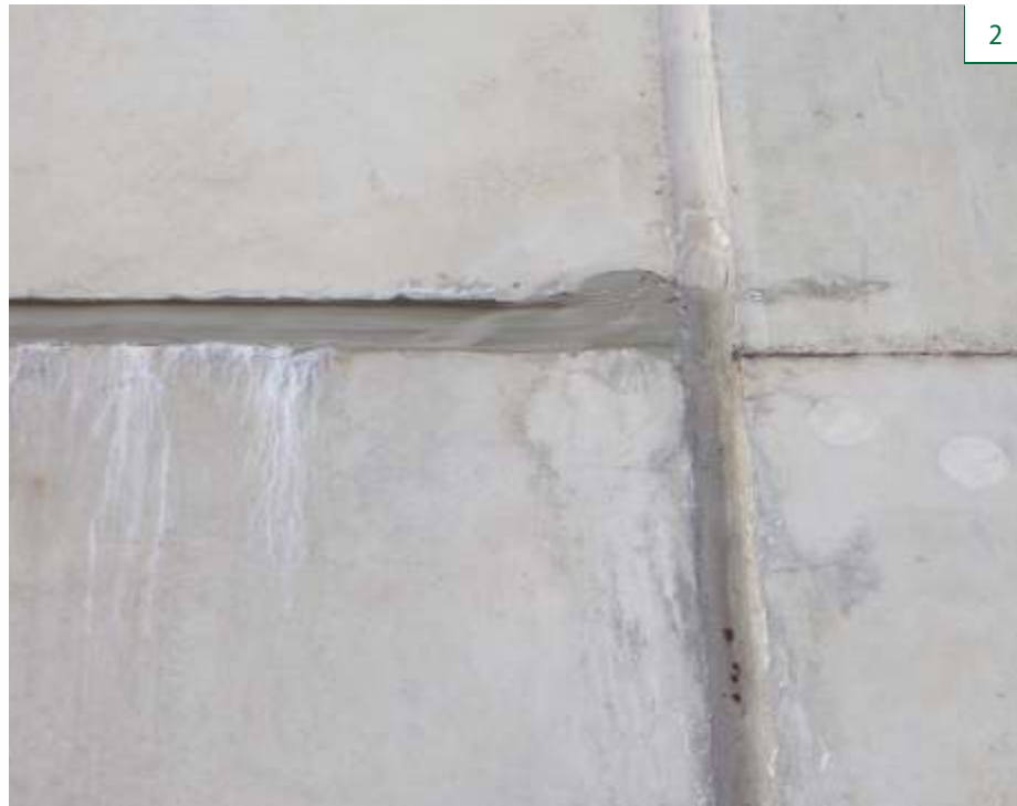
InnoElast® for joint repairing
